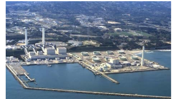
TEPCO Hitachinaka Power Station
